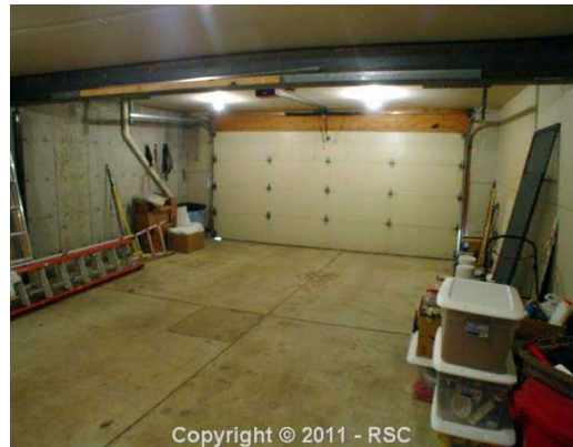
Copyright © 2011 - RSC Garage Interior
